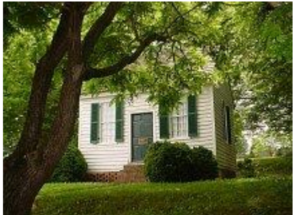
Moved and restored Office on Masonic Street
