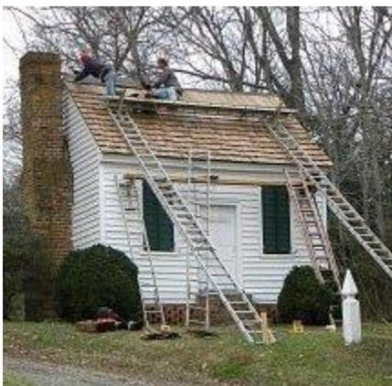
*Roof being replaced with cedar shingles, 2009*
