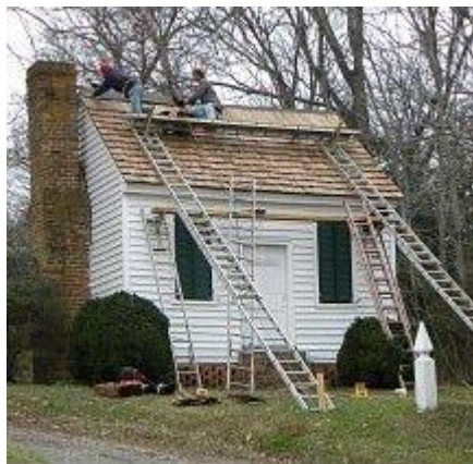
Roof being replaced with cedar shingles
