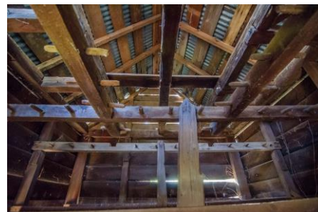
Well-preserved racks and pegs discovered above a lower false ceiling
