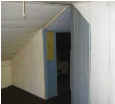
Door into southeast room
