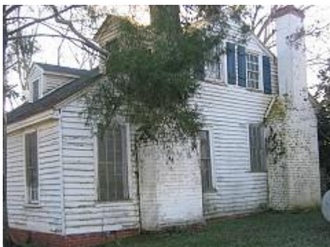
North side, McClenahan House
