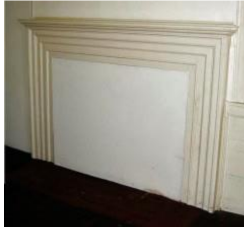
Sealed fireplace in upstairs west room
