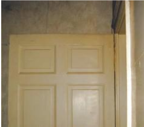
Six-panel door in hall
