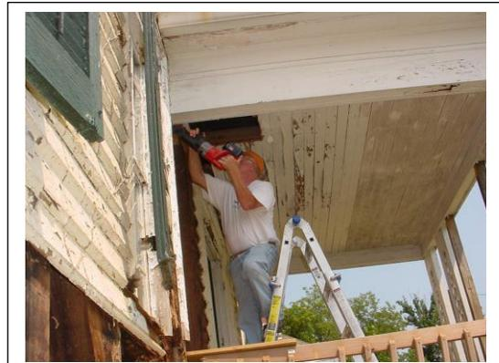
Ray Carney works to stabilize a deteriorated beam in order to lock the double doors.
