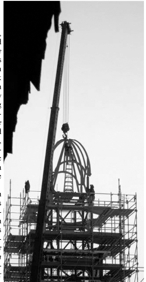
ON NOVEMBER 3, 2012 THE CUPOLA FRAME WAS PLACED.
