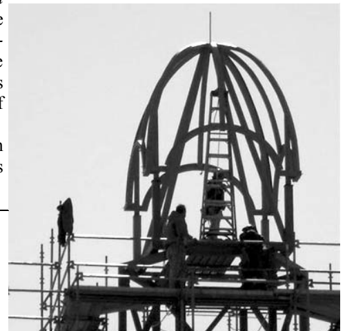
ON NOVEMBER 3, 2012 THE CUPOLA FRAME WAS PLACED.
