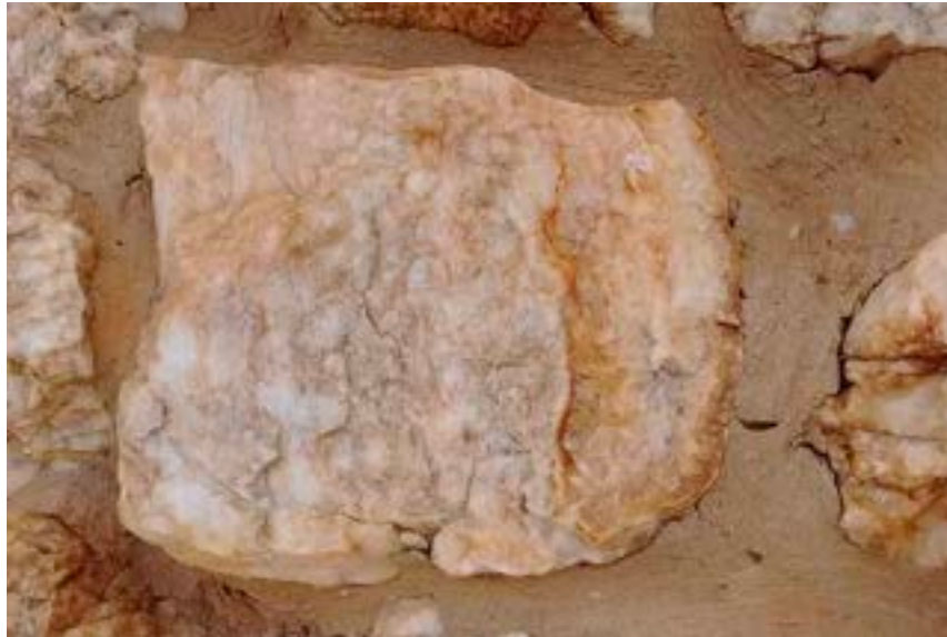
Example of "white flint" boulder used in the "The Rock Store" construction. Note curving and rough surface and iron oxide weathering stains. The "white flint" is a variety of Quartz (Photo credit Asheboro Courier-Tribune ).
