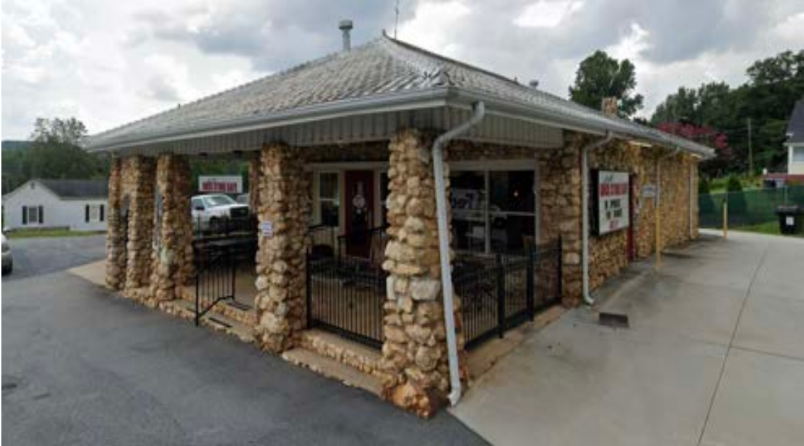
"The Rock Store" located at 1412 Old Liberty Road Asheboro, NC, constructed 1911-1913, an example of using "white flint" for building.
