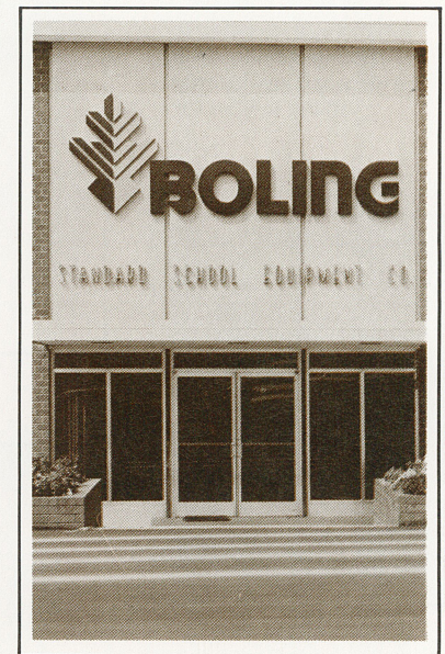
Sign construction workers removed the old Boling Chair Company sign (left) in 1979 to erect a new sign (right) and provide simplified "Boling" identity.
